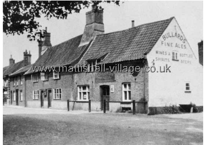
The Swan Inn just before it was demolished in 1932
